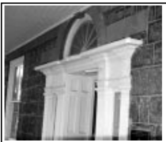
Detail of Main Entrance
