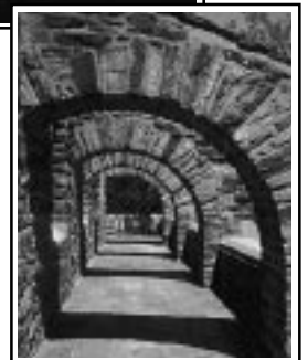
Detail of chapel's buttresses
