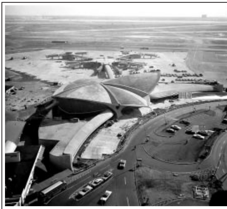
Aerial photograph of the TWA terminal under construction - from the files of the Port Authority of New York and New Jersey.
